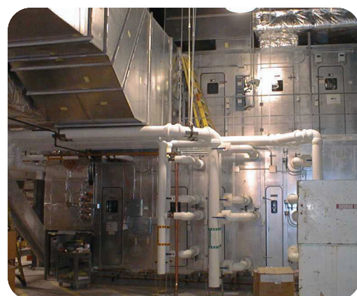
Grunau used two tower cranes to install four custom bi-level air handling units in the six-story addition at St. Luke's Medical Center.
