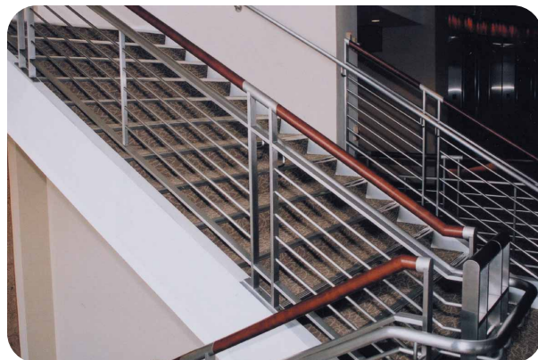
Grunau Metals used a distinct linear polish on all stainless steel railings at Northwestern Mutual's Franklin campus, adding to the architectural quality of the building.
