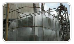
A fire protection discharge test is run at Sammis after the emergency installation of a new transformer.
